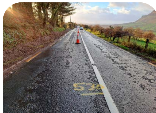
Existing N16 Pavement in Poor Condition
